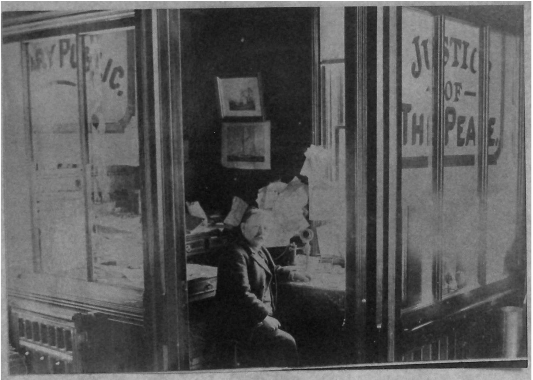
In 1899 Charles Henry Mansfield was in charge of the Western Union Telegraph office, which was located in his store. This photograph shows him in the office. He was also a Notary Public and the Justice of the Peace.
